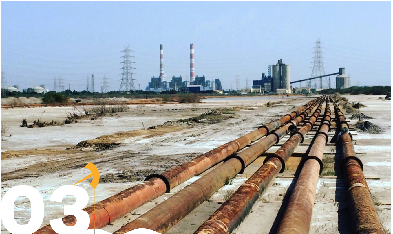
Pipelines carrying coal ash slurry from power plants in Ennore, North Chennai, India
